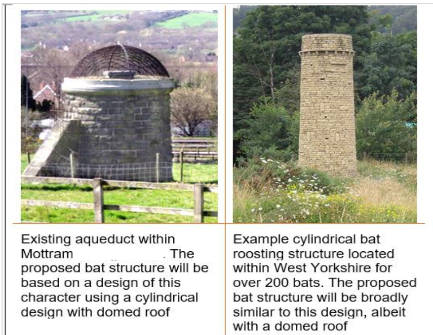
Figure 4-1 Existing natural stone vent structures
